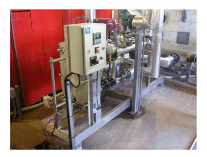
**Customer Requirements:** Replace existing hot water boilers with a packaged heat exchanger to reduce energy costs. Designed around specific existing criteria and restricted footprint.
